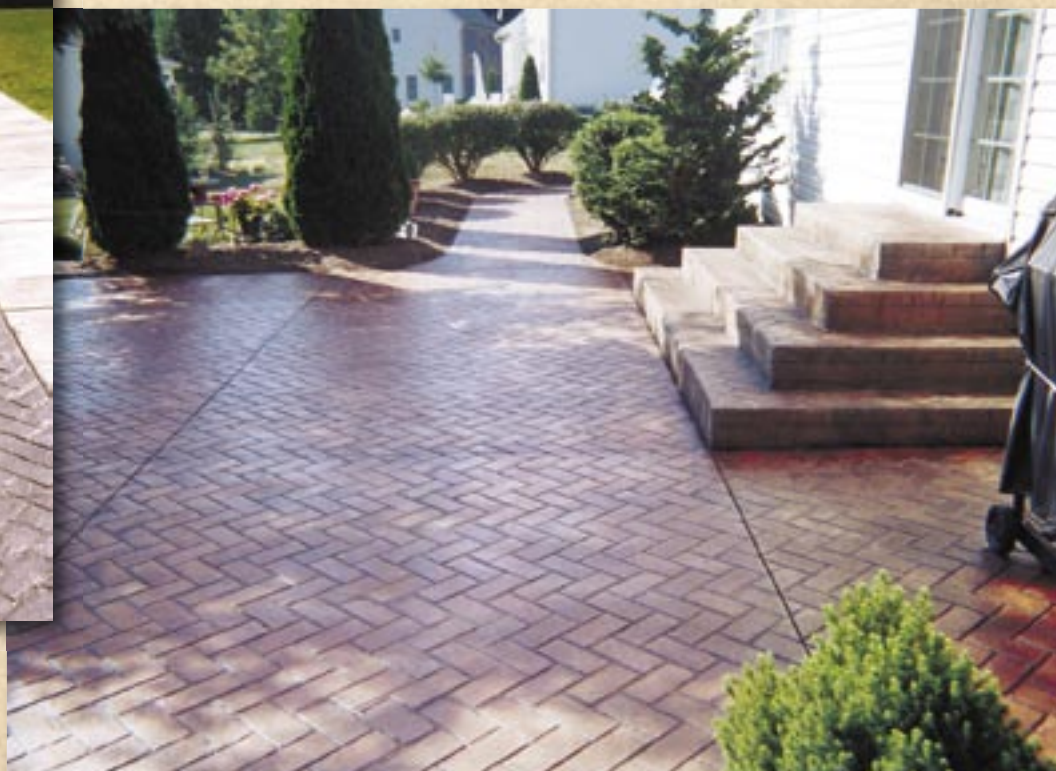
Rust Integral color with Dark Brown Release using a Herringbone Brick design.
