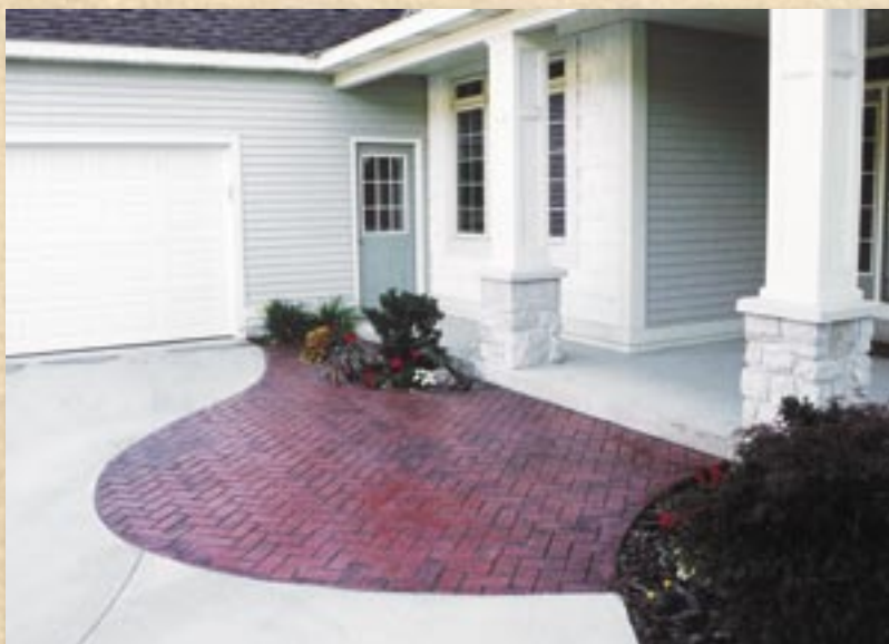
Herringbone Brick using Brick Red Integral color and Charcoal Release.
