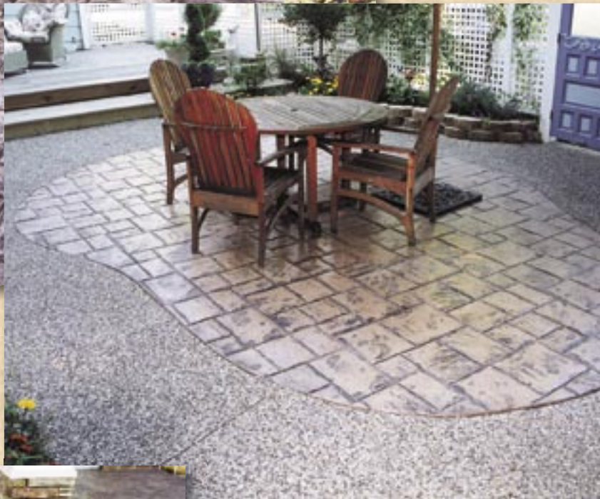
Ashlar Slate using Flagstone Integral color and Charcoal Release.
