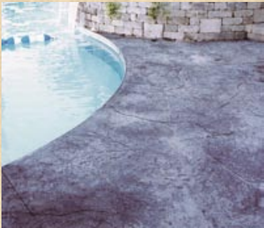
Jumbo Texturing Stone with Silver Integral color and Charcoal Release.
