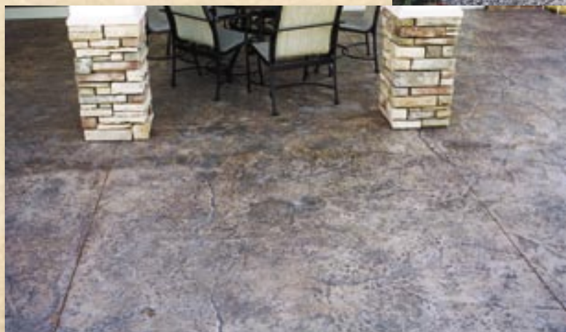
Stone Texturing using Sandstone Integral color and Dark Brown Release.
