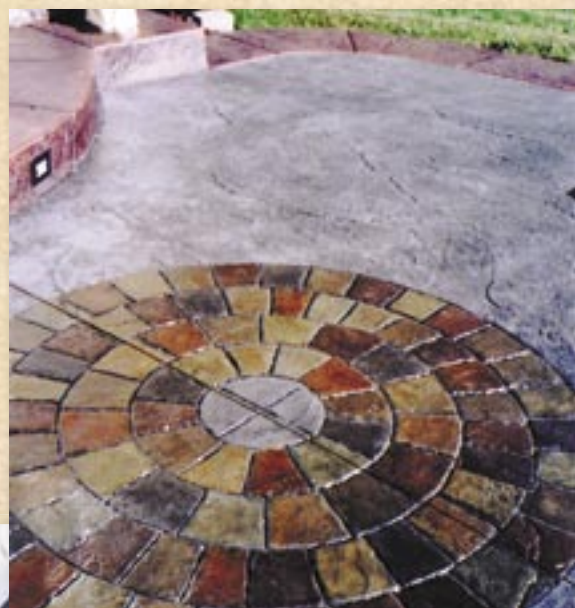
Ashlar Slate design in Sandstone Integral color and highlighted with Brick Red highlighting color.
