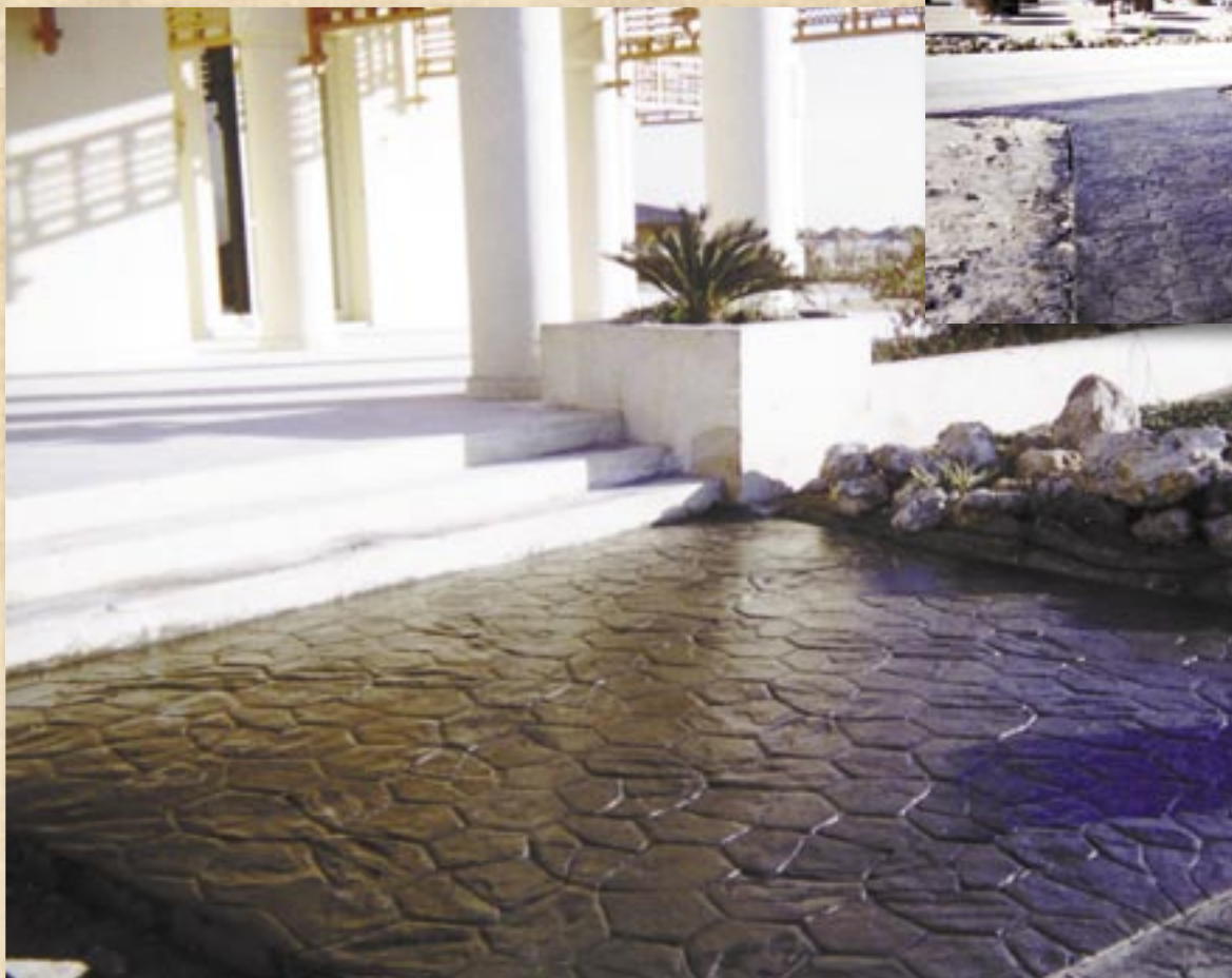
California Fieldstone using Dark Gray Integral color and Charcoal Release.
