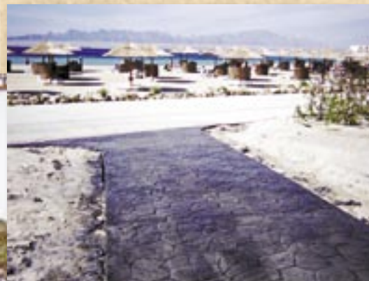
California Fieldstone using Dark Gray Integral color and Charcoal Release.
